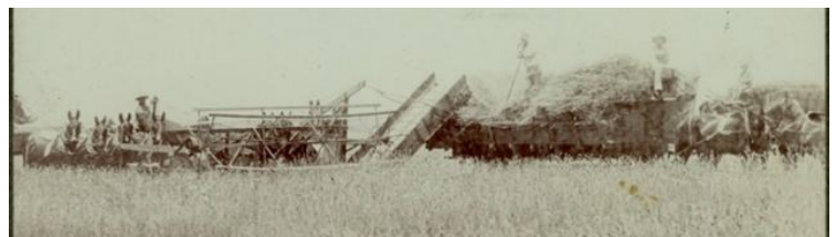
A mowing machine, also called a "header". The horizontal blades gather the cut grain, and it is loaded onto a wagon traveling next to the team via a conveyor belt. Williams photo 1964-12
